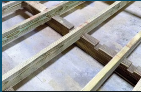
12" On-Center Floor Joists 16" OC is Standard
