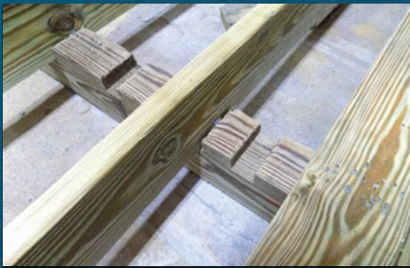
2x6 Pressure Treated Joists 2x4 are Standard
